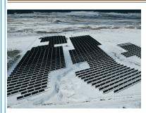
Kit Carson Electric recently completed the 7.5 MW Angel Fire Solar Array which also boasts 3.75 MW of battery storage! This array brings our solar fleet to over 42 MW (40 MW is what's needed to power KCEC's entire daytime electric needs.) In addition, we now have over 16 MW in battery storage capacity.
